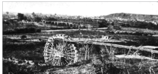
Water wheel built in the 1850s to draw water from the L.A. River. Los Angeles Public Library/Security Pacific Collections.
