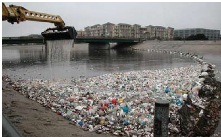
The trash boom at the end of the Los Angeles River in Long Beach. Los Angeles County Department of Public Works.
