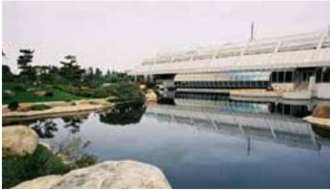
Tillman Water Treatment Facility Los Angeles River
