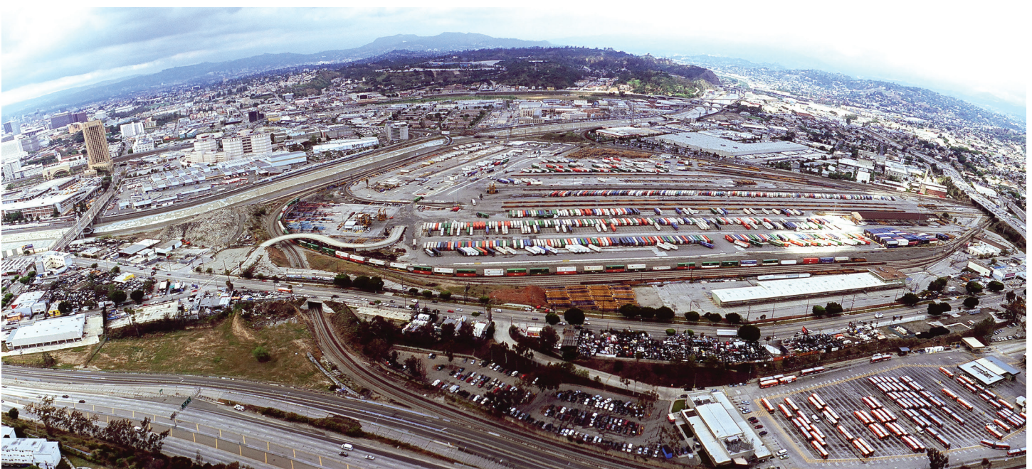
Bird's-eye view of the Piggyback Yard site, also known as the Los Angeles Transportation Center, Source: Ben Feldmann
