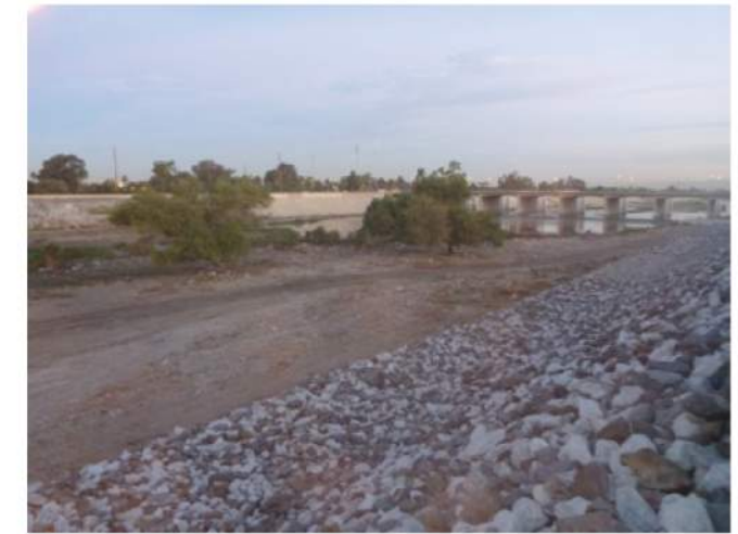
Looking upstream to Willow Ave. Bridge from bike path access ramp
