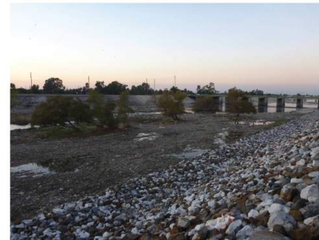
Looking upstream to Willow Street Bridge from bike path access ramp
