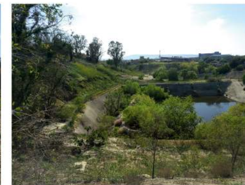
Retention basin captures runoff from 405 freeway.
